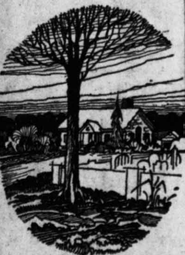
The Crooked Run Baptist Church now pre-empt's the site of the missing Bethesda auf der Morvan — Lutheran edifice.
